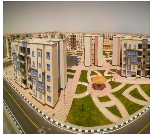
Figure 9: Social Housing Project Units (2012-2017)
